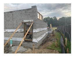
FD- Block out installation for future glass block, louver, and roll up doors
